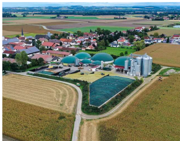
Biogasanlage in Oberindling.
