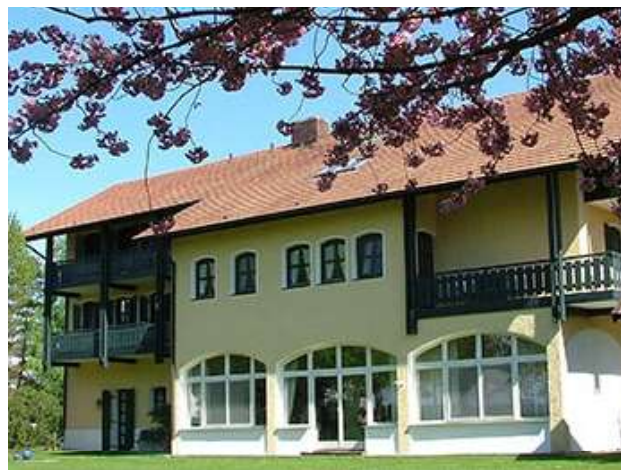
Apartmenthaus in Pfaffing.
